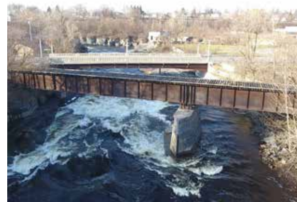
The former rail bridge on the west side of Sewall's Island.
