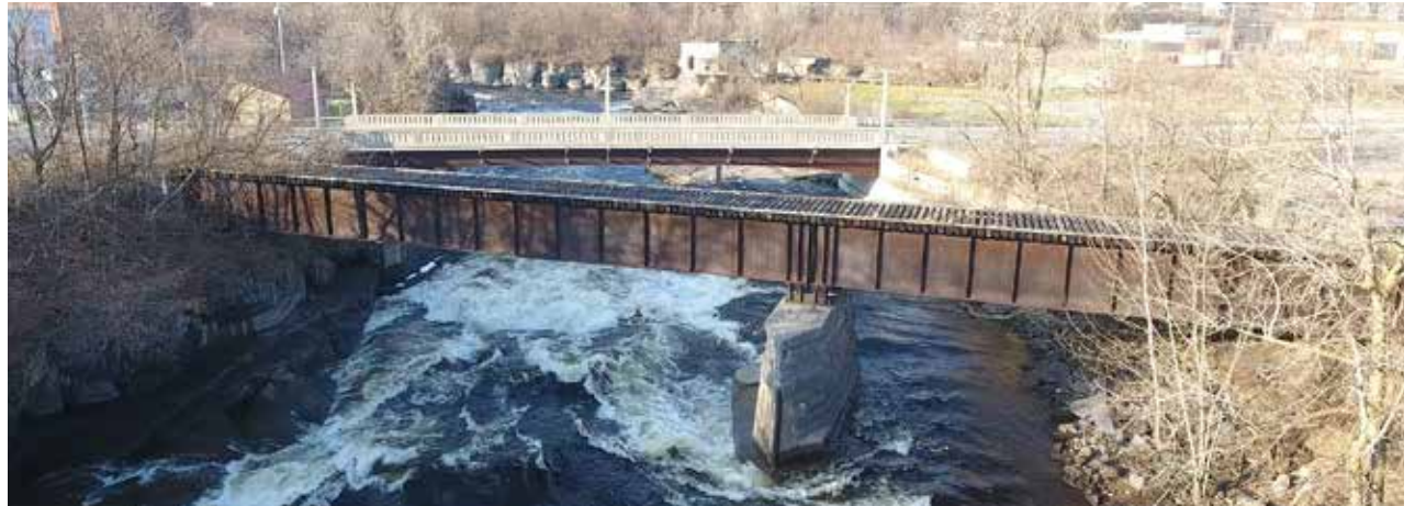
The former rail bridge on the western side of the island crosses over rapids in the Black River.
