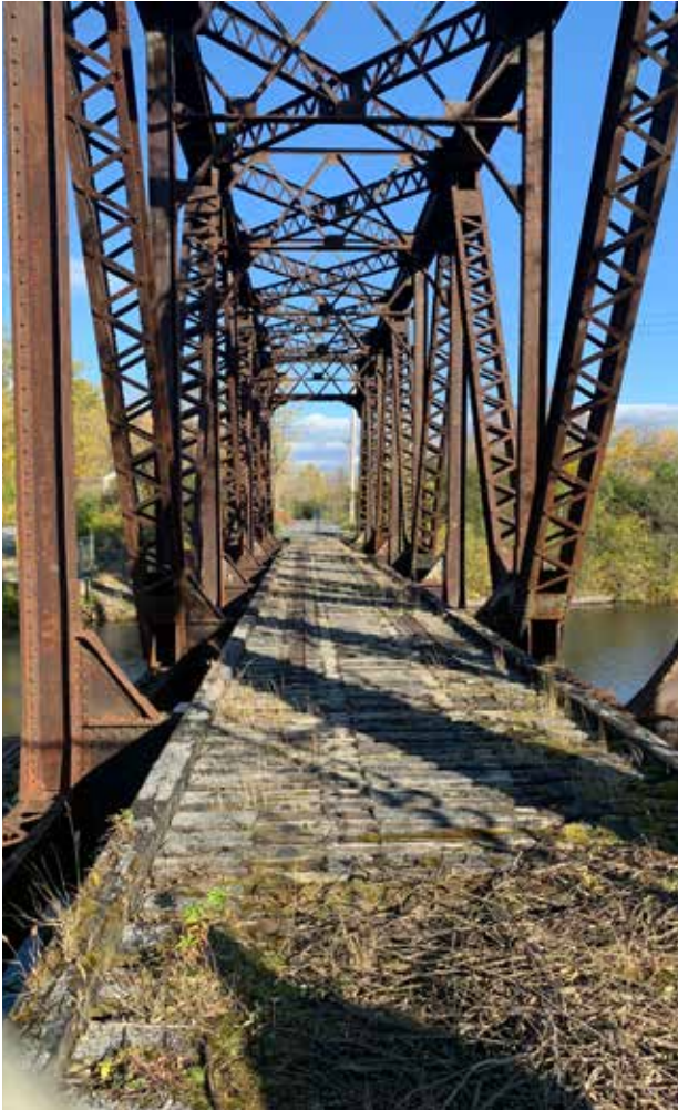
The former rail bridge on the east side of the island.
