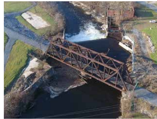
The former rail bridge on the east side of Sewall's Island.
