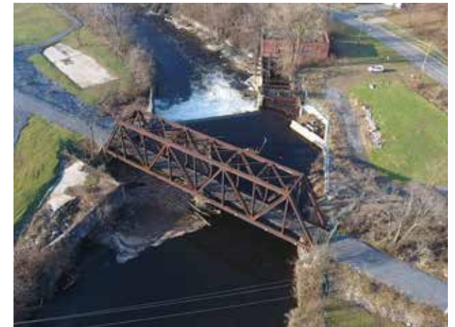
The bridge on the east side of Sewall's Island is another incredible historic asset for the plan.
