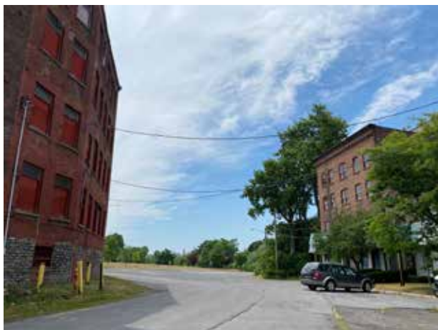
The existing buildings offer opportunities for reuse.
